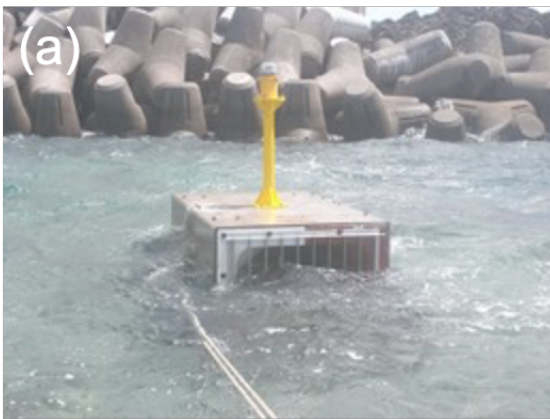
Figure 2. The Taper-Ducted OIST Wave Energy Converter device during the installation (a) and during operation against a breaking wave (b). A yellow LED beacon is installed on top of the structure and metal frame is installed on the inlet of the Duct for safety reasons.
