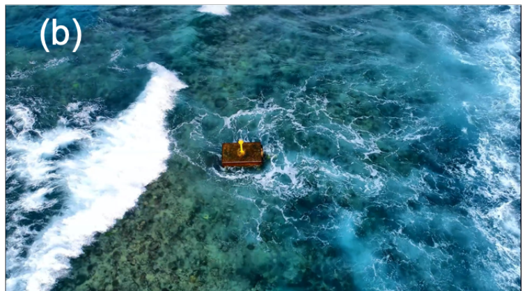
Figure 2. The Taper-Ducted OIST Wave Energy Converter device during the installation (a) and during operation against a breaking wave (b). A yellow LED beacon is installed on top of the structure and metal frame is installed on the inlet of the Duct for safety reasons.
