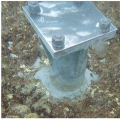
Fig. 5. After drilling the holes, we inserted the sockets, and filled the gap with ceramic-balls, then sealed with epoxy cement on the top. Then we mounted the WEC support, by inserting it into the socket. The square block in the bottom left photo is the zinc anode to reduce rusting.
