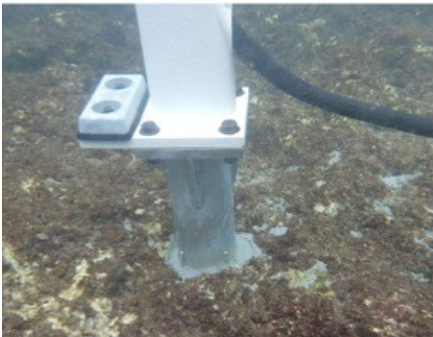
Fig. 5. After drilling the holes, we inserted the sockets, and filled the gap with ceramic-balls, then sealed with epoxy cement on the top. Then we mounted the WEC support, by inserting it into the socket. The square block in the bottom left photo is the zinc anode to reduce rusting.
