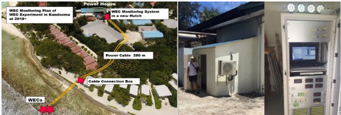
Fig. 10. Power monitoring system and power cables. | Fig. 11. Power monitoring shed and monitoring system.
